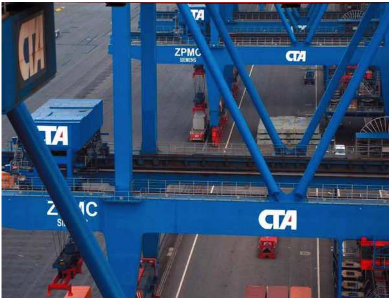
An igus® energy supply system with a length of approx. 26 m in a stainless steel trough with middle band support.
