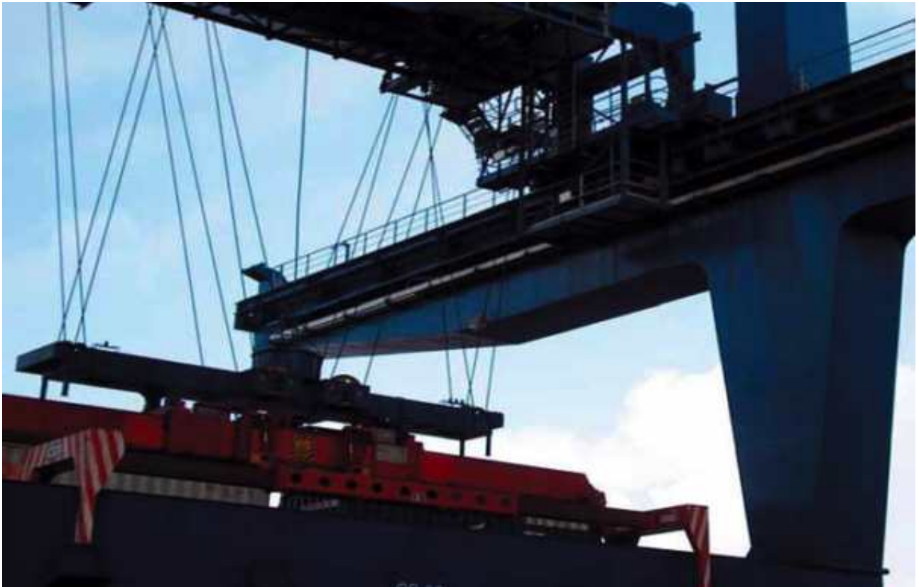
The Energy Chain System® was filled with many different igus® Chainflex® cables, e.g. the CF9.60.05
