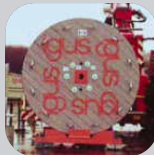
Crane travel up to 100 m, assembling from the roll.
